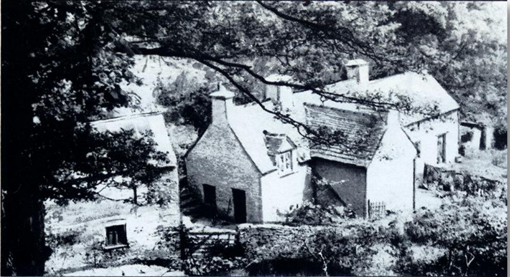
View of Pandy Cottages
